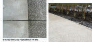
PAVED SPACES PEDESTRIAN PATHS: Saw-cut broom finish concrete (entry profile) and 100mm wide saw-cut exposed aggregate concrete (edge detail) PAVED COURSEDS: Aggreg to curbside dual parking kerb for an additional edge setting to minimise excavations and disturbance
